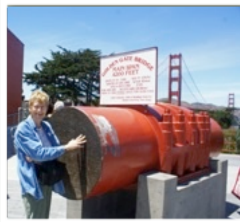
Betsy Gottshall standing beside a sample of the cable used to support the Golden Gate Bridge.
